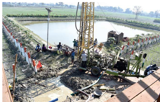
Fig. 12.2. Water storage pond and installation of borewell
