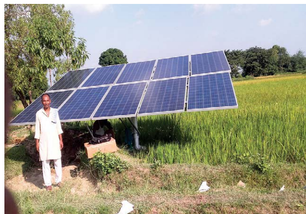
Fig. 17.4. 3HP-3000 Wp Solar groundwater pumping systems in Bhagwatipur village of Madhubani district of Bihar
