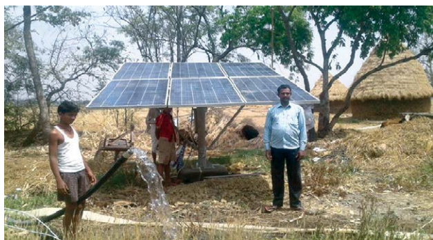
Fig. 17.3. 2HP-1800 Wp Solar water pumping system in Bharatpura village, Paliganj block of Patna district.
