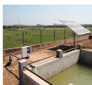
Fig 16.2. Solar pumps, operated by 3.0 kWp solar array, selected for evaluation in eastern region
