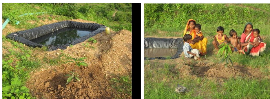
Fig. 6 Doba: a small water harvesting tank for uplands
