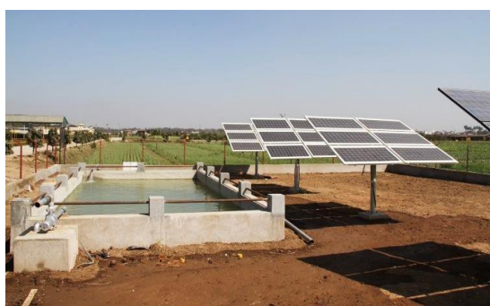
Fig 1: Solar photovoltaic groundwater pumping system model for small farms.
