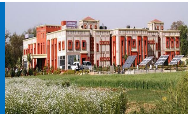
Administrative building cum Laboratory, ICAR- RCER, Patna
